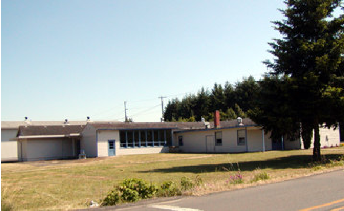
Fairview School as it looks today. Since its closure it has been used as a church.
